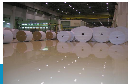
ROMEX® industrial floor coating for the use of air cushion transport systems in the paper and foil industry
