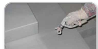
Can also be applied using airless spray method
